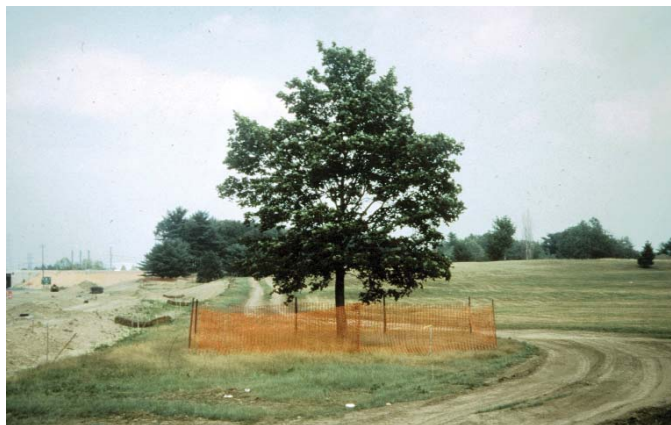
Figure 4. Save as many trees as possible on land under development. Protect trees during construction.
